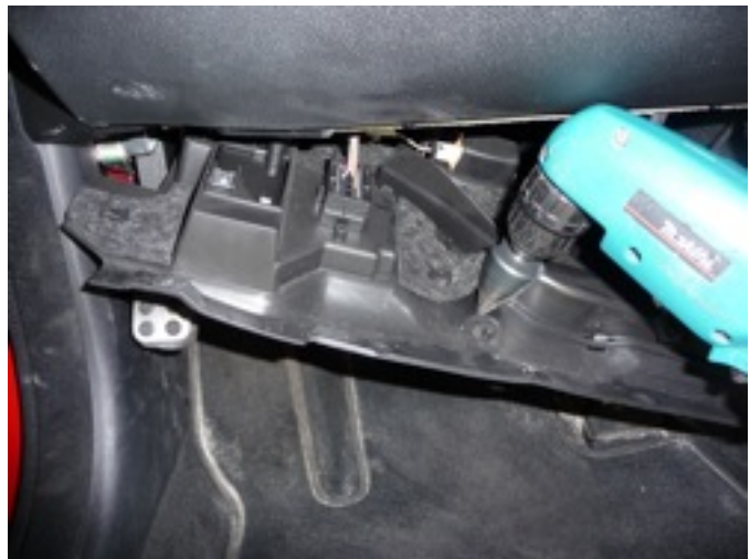
Drill valet switch hole in under dash panel
