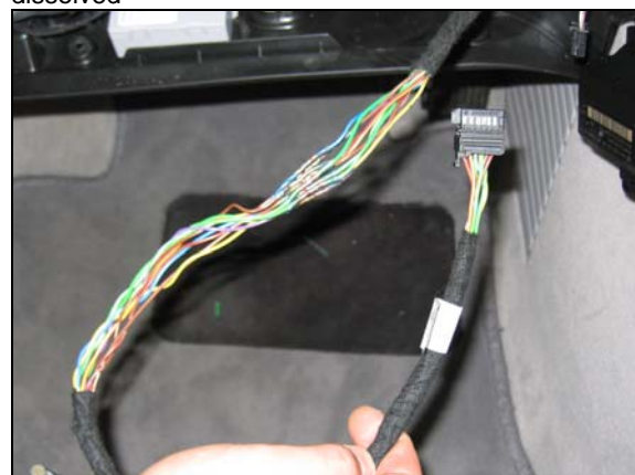
Figure 8 P-B-91.60/99c Repair harness spliced to vehicle harness (Repair as of MY 05)
