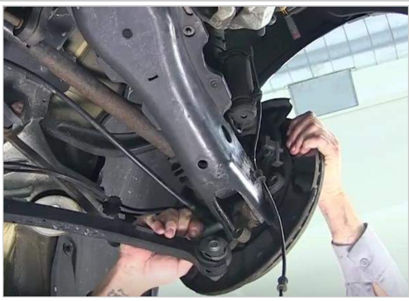
Removing spring control arm to wheel carrier bolted connection.
