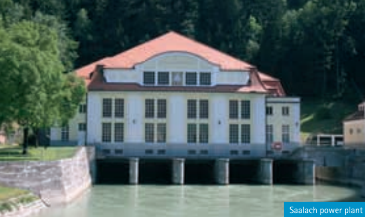
Saalach power plant
