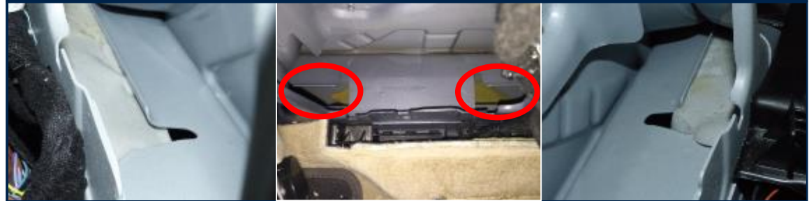
Foam piece installed
