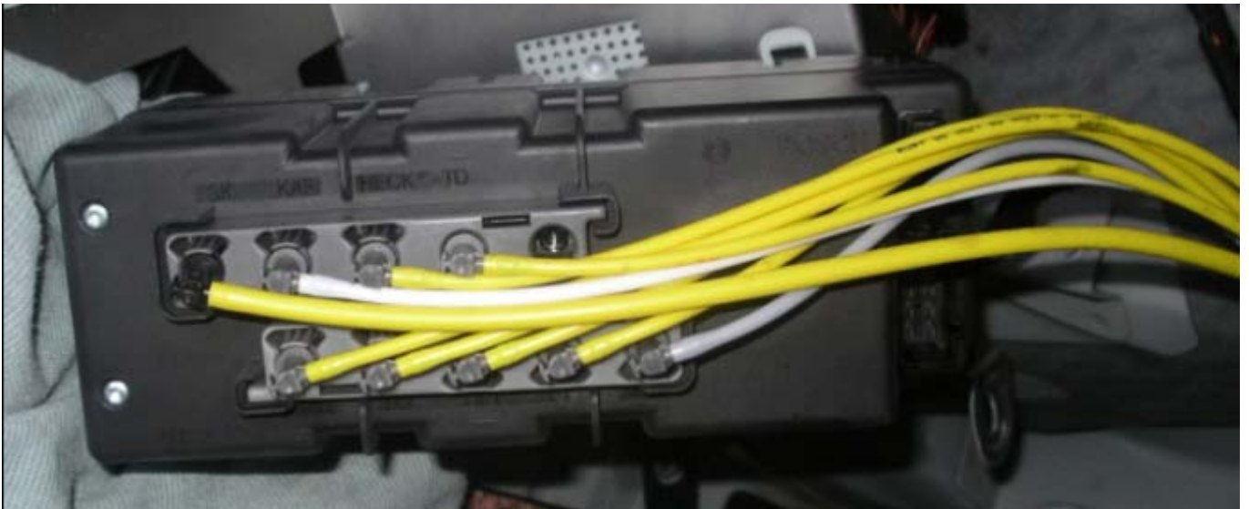
Figure 1 MB OEM Pneumatic System Equipment (PSE) Pump in Boot/Trunk
