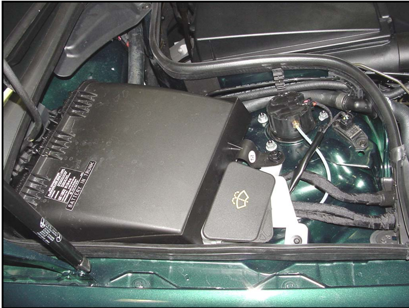
Auxiliary battery installed below air intake of HVAC
