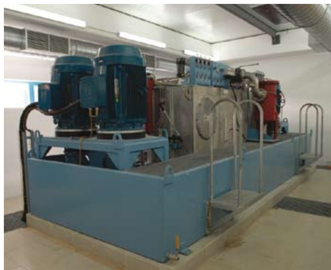
The aggregates for the Leixoes bascule bridge are driven with RENOLIN B10 hydraulic oil.
