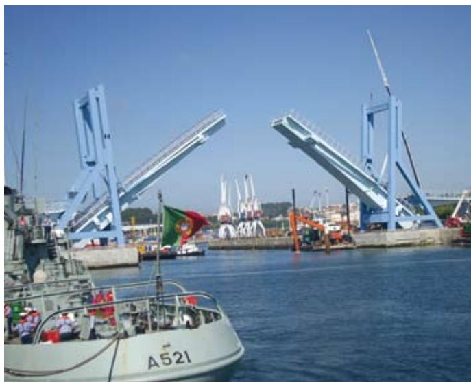
The new bascule bridge in Leixoes harbor is one of the most spectacular constructions of its kind.
